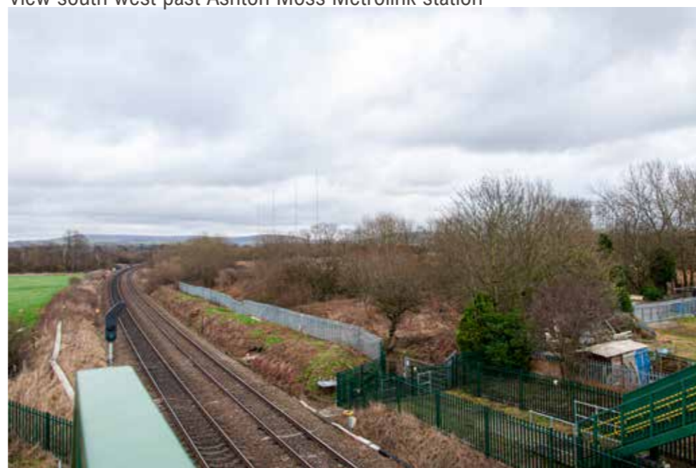
View of railway line to the north of the site, looking east from pedestrian railway bridge
