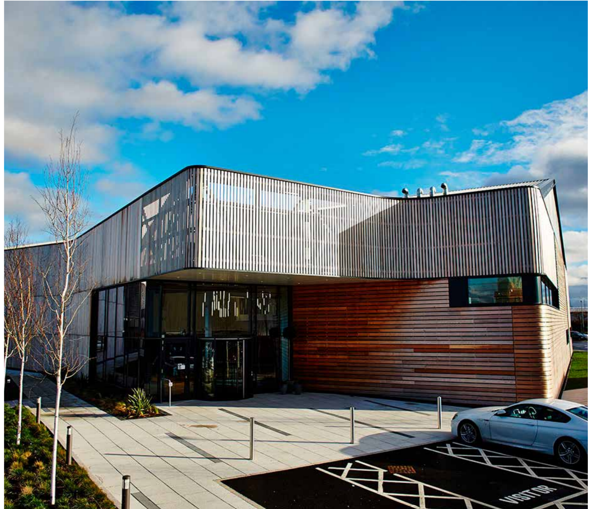
Regatta Building, Trafford, Manchester
